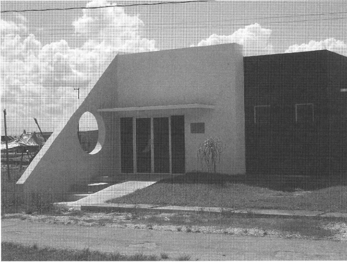
Figure 3b : Nursing home in Peto built by the Tres por Uno program yet to function (May 27, 2007, photo by the author)
